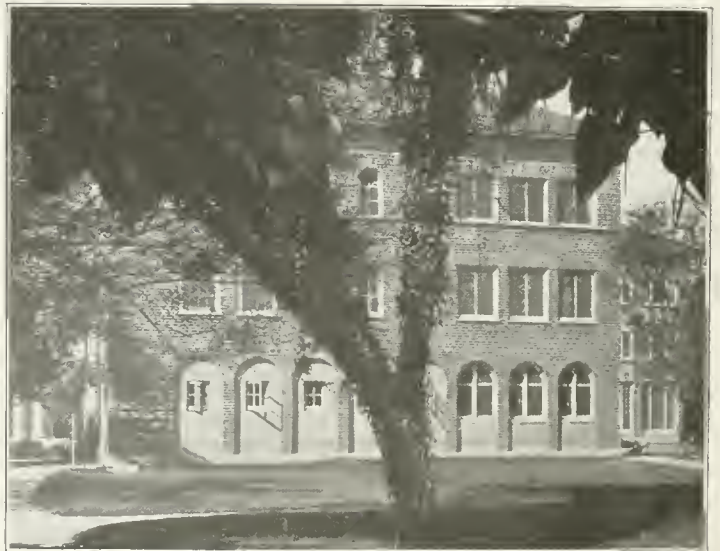
Exterior view of Maricopa Hall, women's dormitory. A good view is given of opening for sleeping porches on three floors
